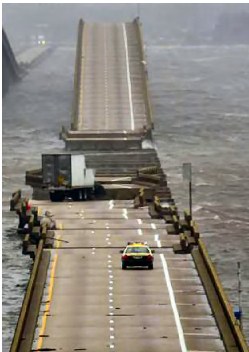
F-3 | SECTION OF AN INTERSTATE 10 BRIDGE OVER ESCAMBIA BAY, IN PENSACOLA, FL, WASHED OUT DURING HURRICANE IVAN
