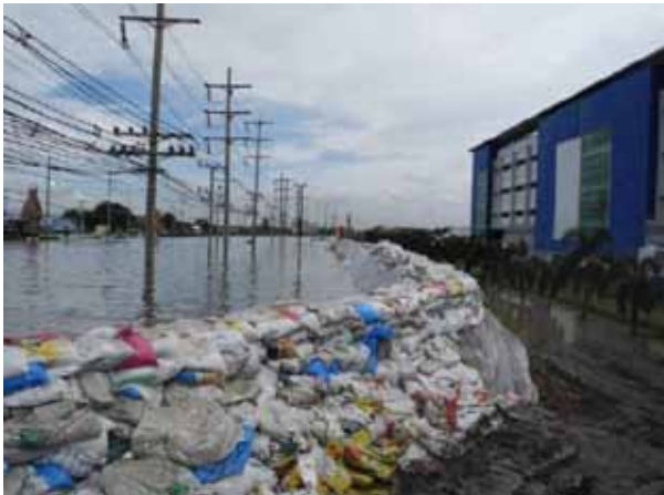
Bang Pa-in industrial park before breach
