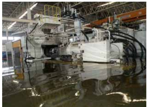
Damage to machinery due to flooding
