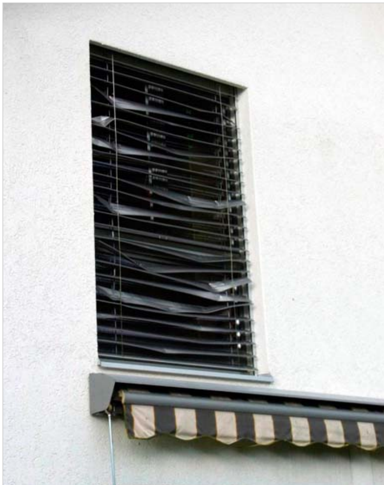
Figure 11: Blind damage at a home in Tentlingen, Fribourg Canton, following the hailstorms
