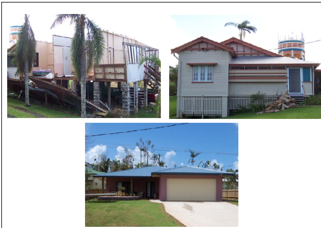
Figure 3: The different building standards were very evident in Innisfail
